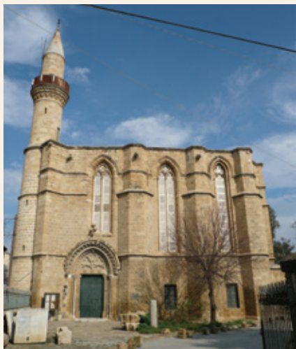
1 The church of Saint Catherine (14th century) in the occupied city of Nicosia, within the city walls, is very close to the Cathedral of Saint Sophia. It is an elegant church built according to the standards of southern France and one of the most important Gothic monuments of Nicosia.
