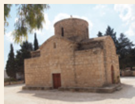
4 Photos of the church of Panagia Chortakiotissa from the non-surviving homonymous monastery in the area of Frennaros-Sotira. The first photo is from 1945 and the second photo illustrates the church today, after the maintenance works and the reshaping of the area.
